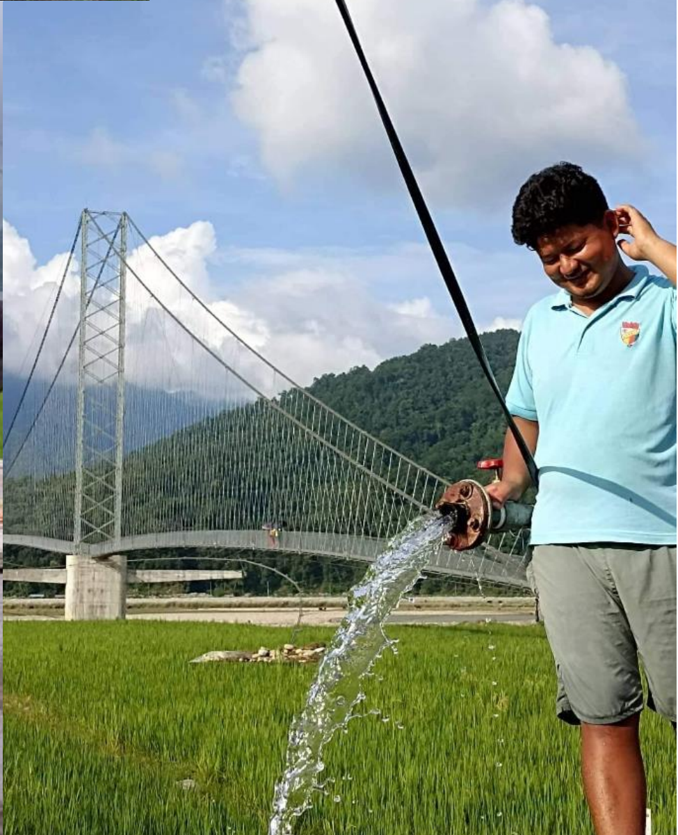
Installation of solar pump to lift drinking water
