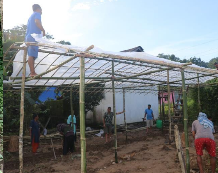
Project beneficiaries constructing a poly-house tunnel for commercial vegetable farming
