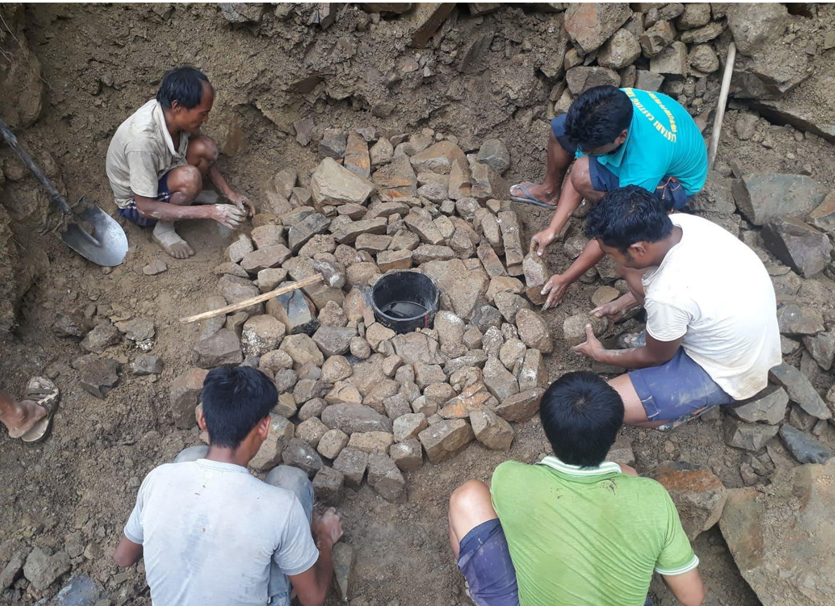
Local Beneficiary Contribution in Laying Foundation for the Forebay
