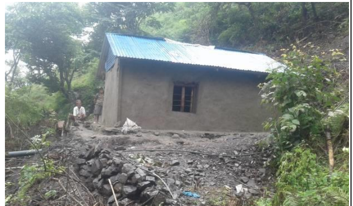
Constructed Power House of IWME
