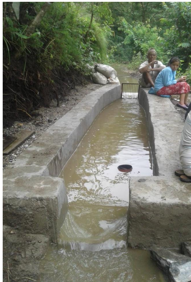
Constructed Intake and Canals IWME
