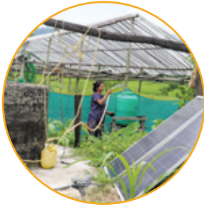
Kanchi Maya using portable solar pump to lift water from newly rehabilitated well
