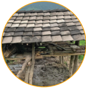
Unmanaged cow shed
