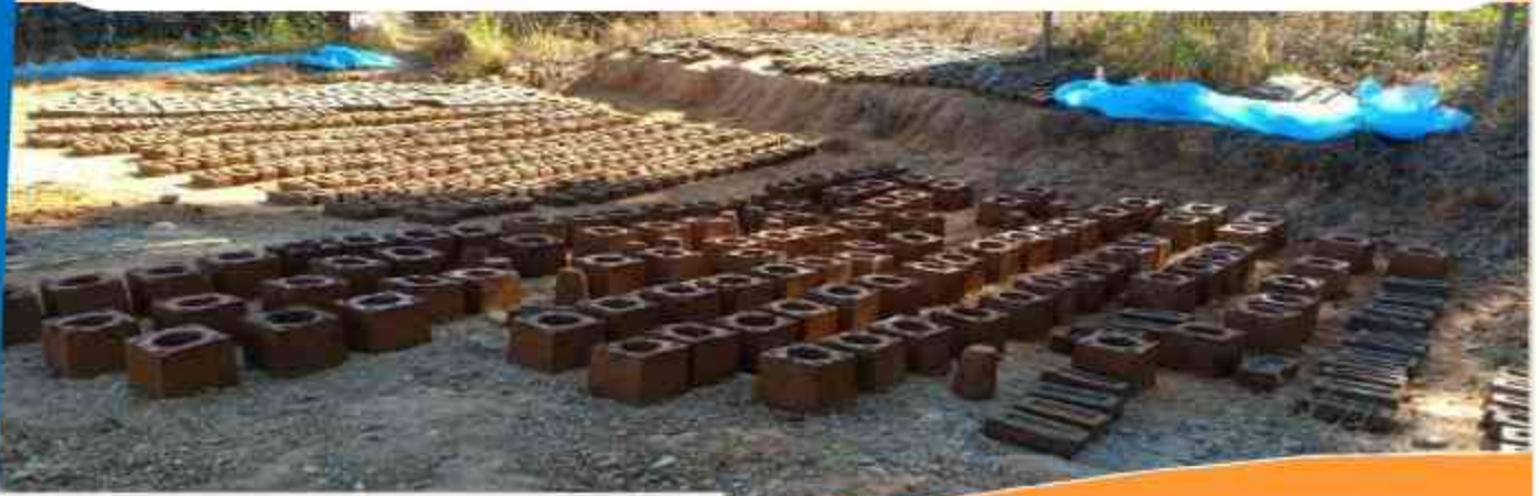
Prepared Bricks & Chimney by Participants
