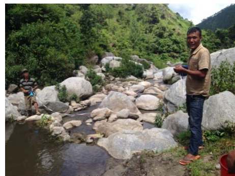
Figure 4 Survey for construction of canal for powerhouse
