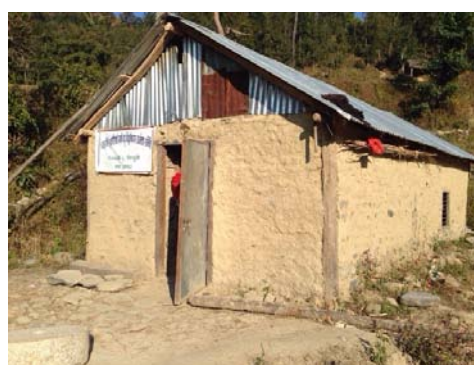
Figure 6 Powerhouse of Barabise IWME Project
